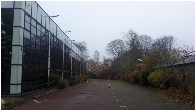
South elevation & boundary
